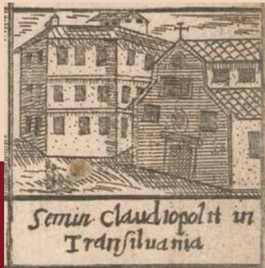
The church of the Major Jesuit College of Cluj and the building that is supposed to have hosted the Gymnasium, the Pontifical and Royal Seminary, and the Academia Claudiopolitana .
